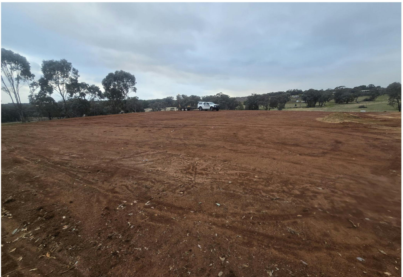
Site Photo 1 – Looking South-West (10/07/2025)
